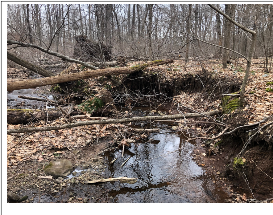
Photo 2: View of eroded stream bank south of crossing #1
