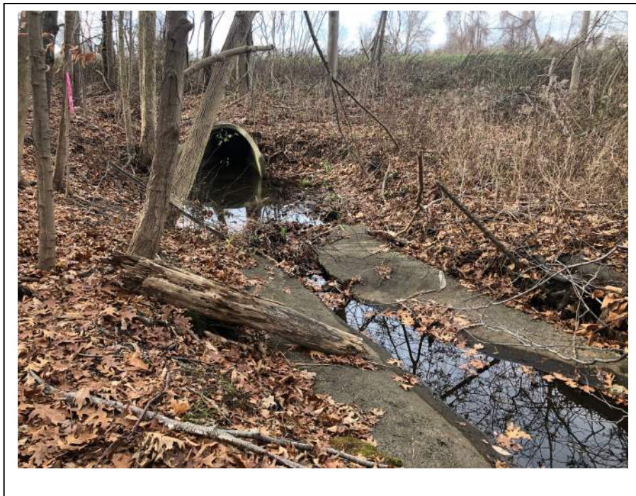
Photo 4: View of point of origin of the intermittent watercourse upgradient of crossing #2. Interstate 91 is in background. Note concrete bed.
