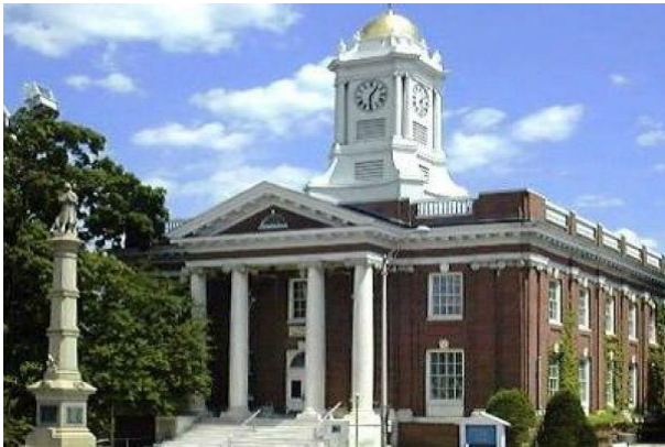
City Hall, Meriden CT
