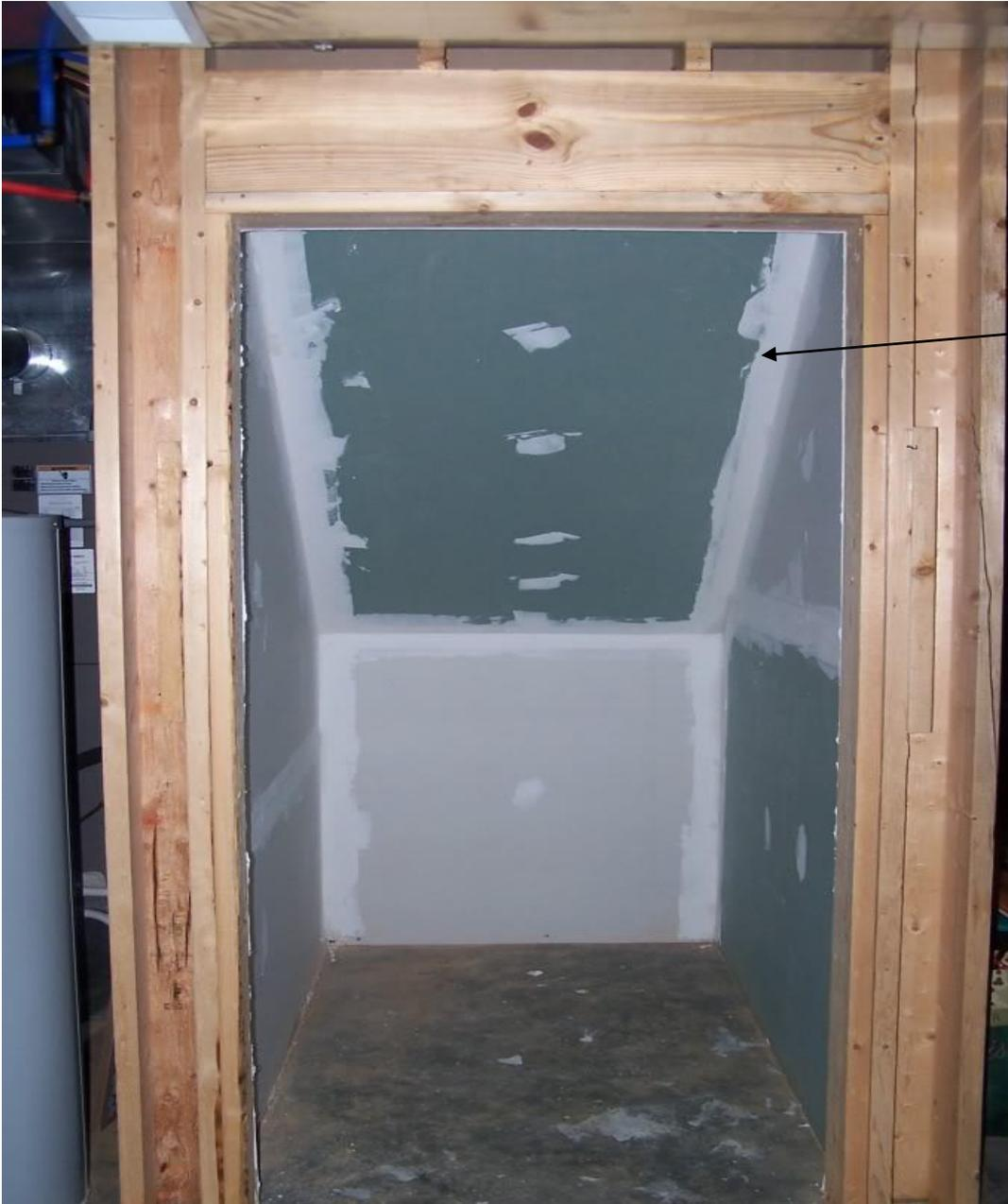
Drywall required on the underside of basement stairs when a closet/storage is being added.
