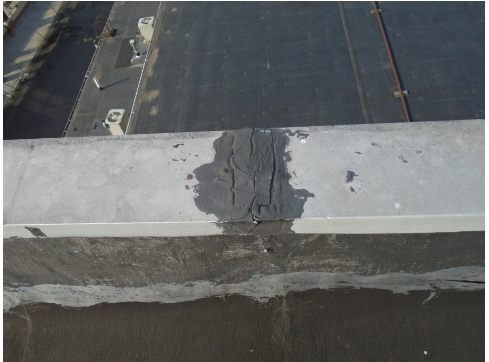
Photo P7 Tarred over coping joint.
