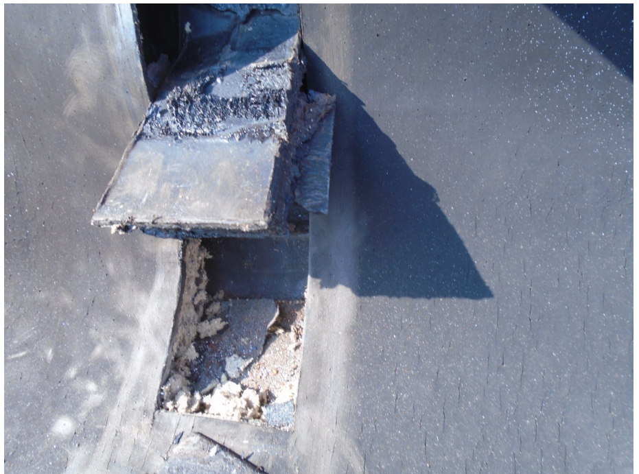
Photo 13 Photo of Test Cut #4 close up.
