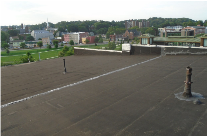
Photo P2 General view looking southeast
