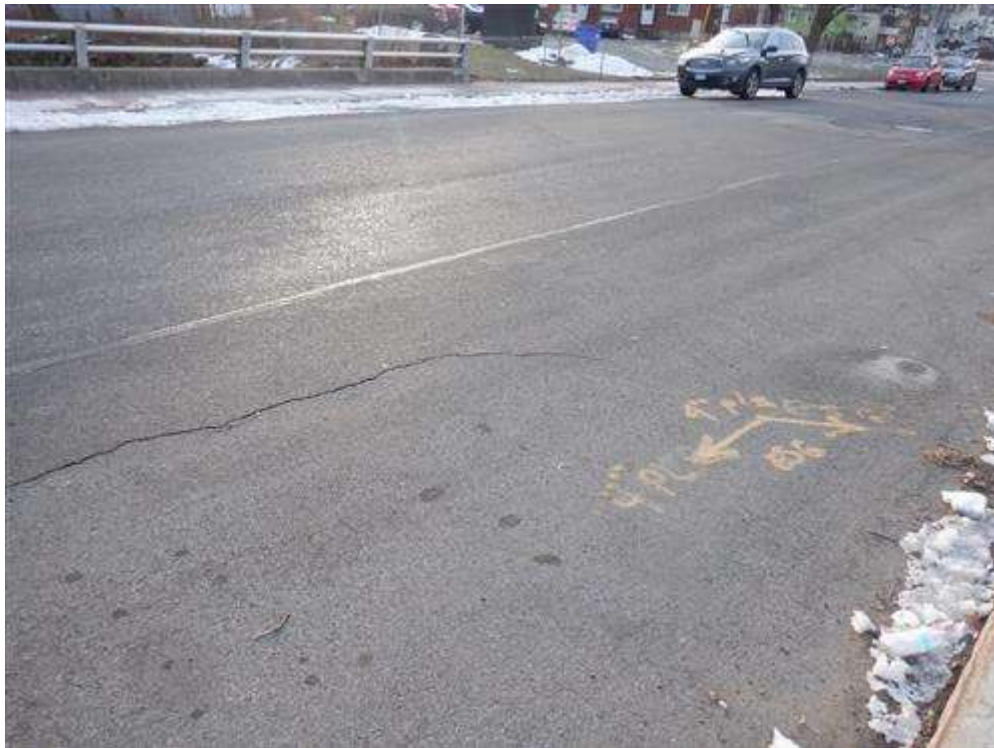
Typical condition of the bituminous pavement over the bridge. Note the longitudinal crack extending from the approach pavement.
