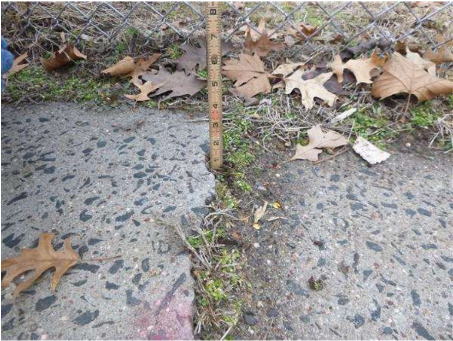
Vertical misalignment along the southeast approach sidewalk (due to crack), at the 1st approach sidewalk panel from the bridge.
