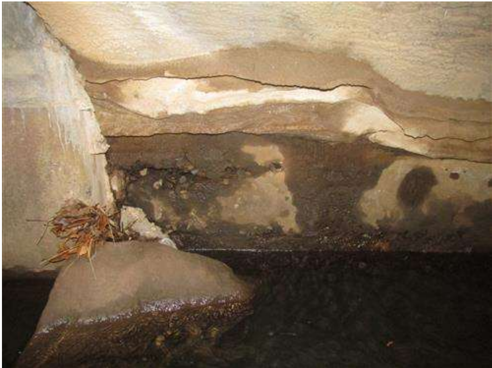
Abutment 2 at the west end has scaling.
