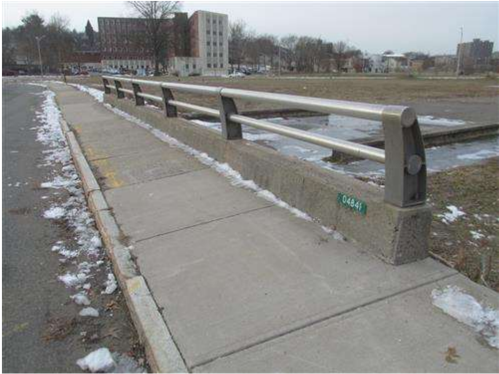
West curb, sidewalk, rail base and railing.
