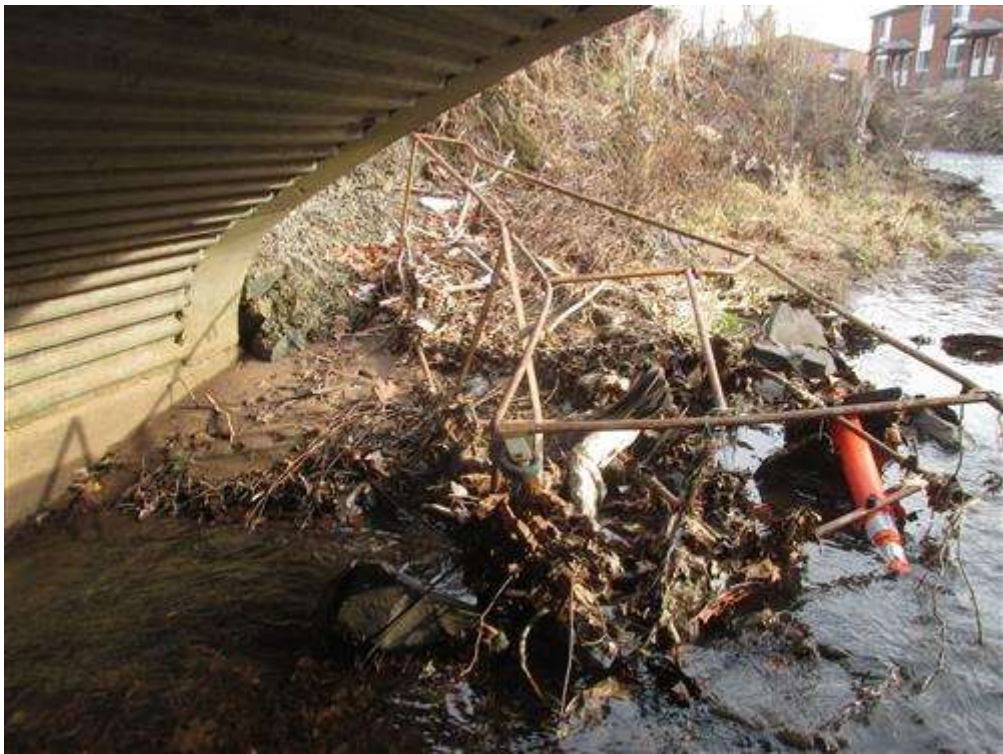
Accumulation of debris at the east end of Abutment 2.
