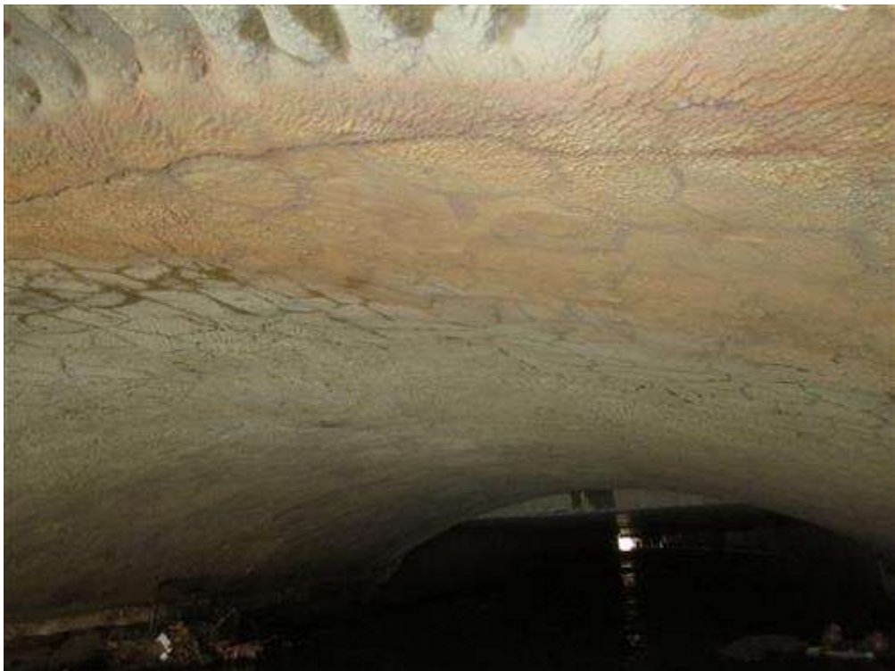
Typical condition of the old concrete arch underside.
