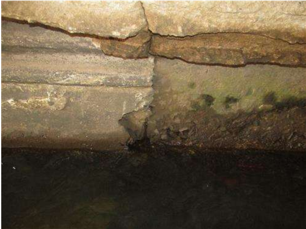
Abutment 1 along the joint between the older and newer concrete arch sections has a void.
