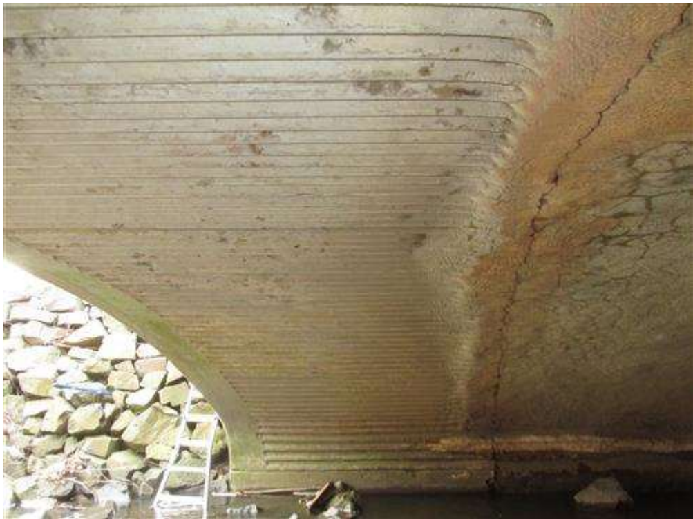
Typical condition of the new concrete arch underside.
