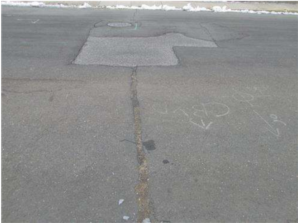
Pavement at Abutment 1 has a transverse crack and a patch.
