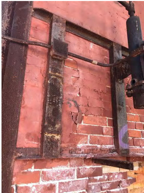
Red coating on brick of boilers
