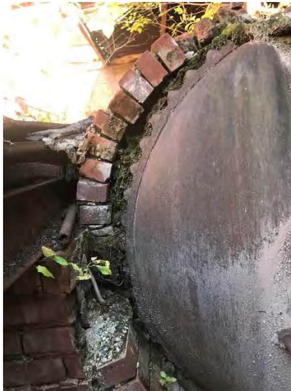
Photo showing degradation of tank insulation
