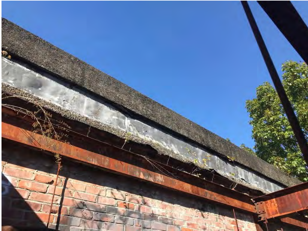
Roof flashing remaining on parapet wall after roof field has collapsed
