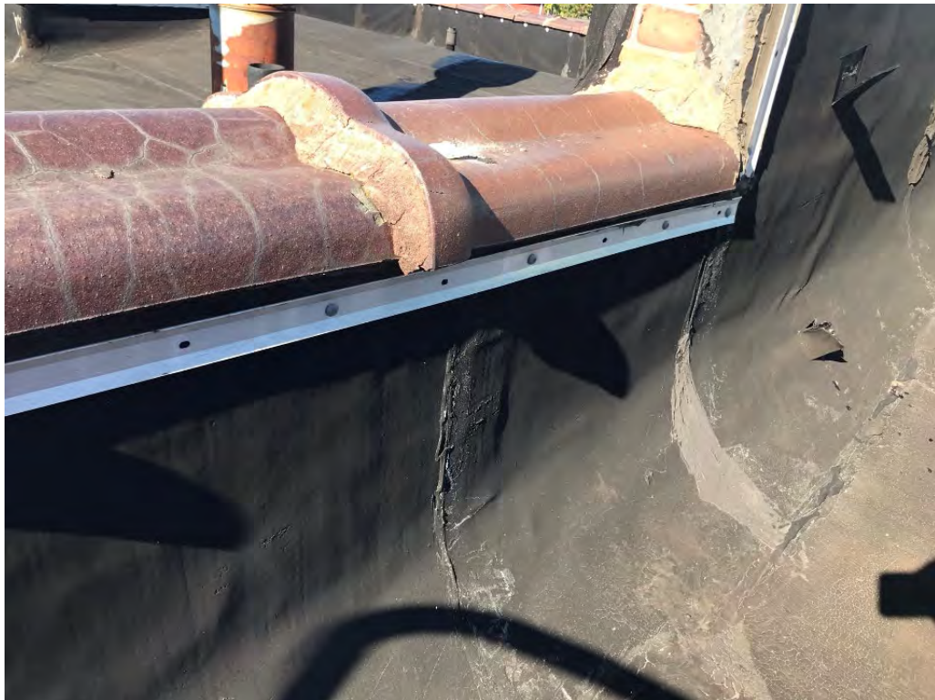
Main building roof metal flashing (termination bar) caulking
