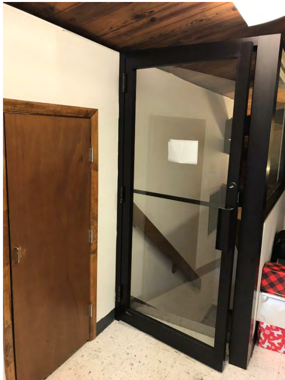
Type 12 Door (Right): No caulking or glazing observed
