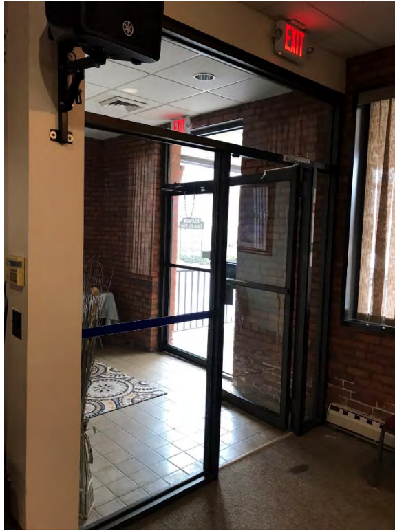
Type 5 Door: Dark Gray Caulking; Non asbestos, Presumed PCBs >50 PPM (same caulking as Type 3 Door); No glazing observed
