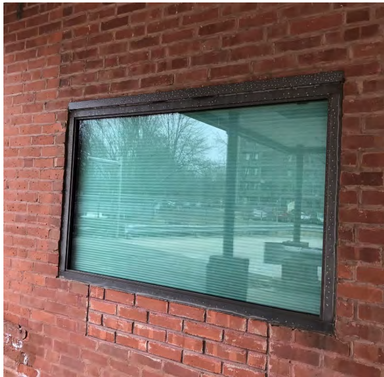
Type 5 Windows: Brown Caulking: Non asbestos, Presumed PCBs >50 PPM; No glazing observed
