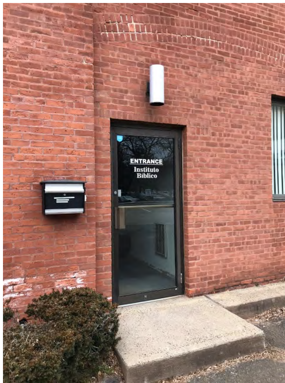
Type 4 Door: Light brown caulking: Non asbestos, Presumed PCBs >50 PPM; No glazing observed
