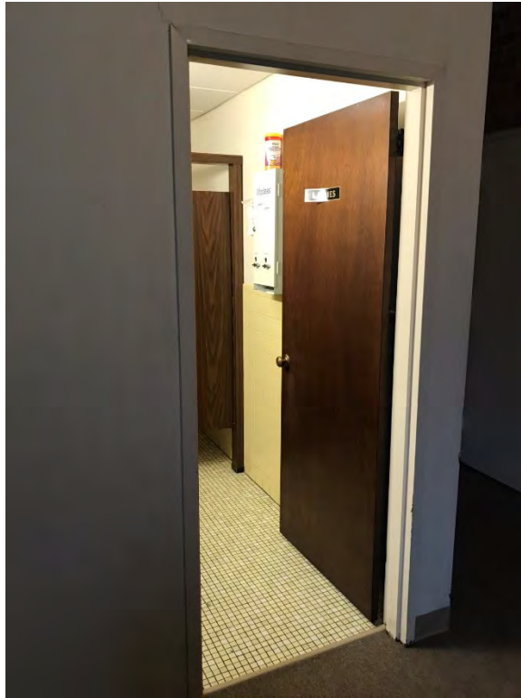
Type 9 Door: No caulking observed
