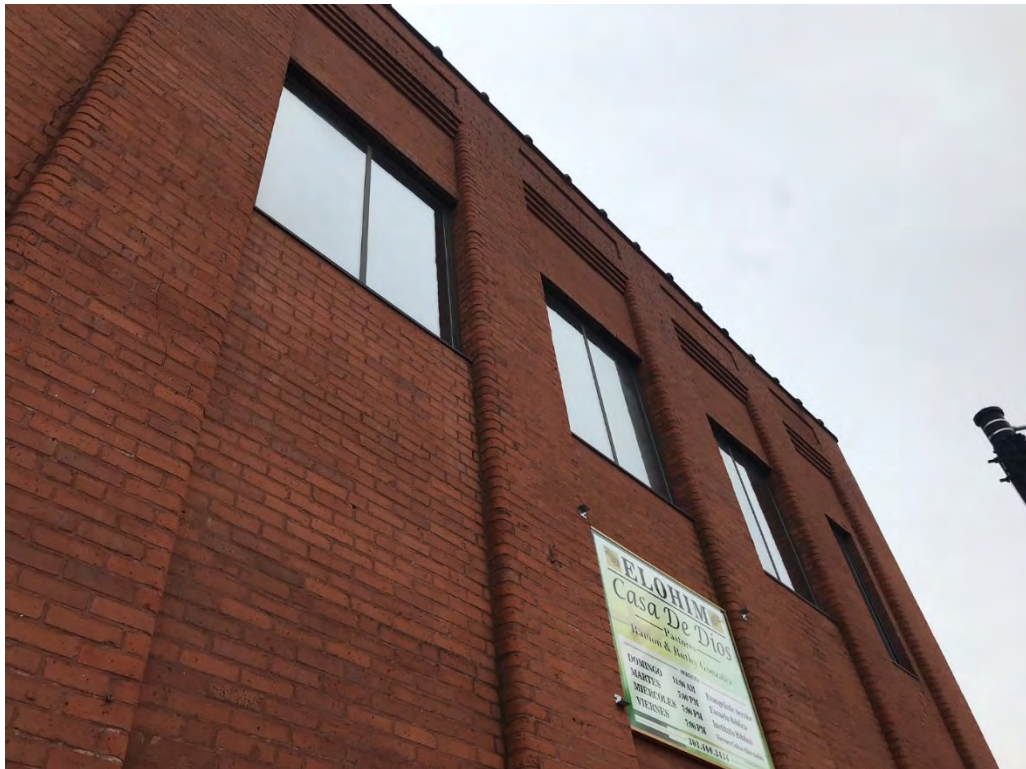
Type 2 Window: Gray caulking: Non asbestos, Presumed PCBs >50 PPM; No glazing observed
