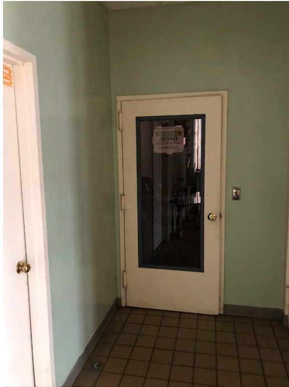
Type 7 Door: No caulking; Light gray glazing: Presumed PCBs >50 PPM
