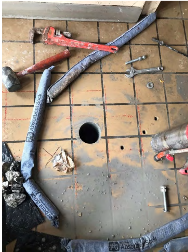
Concrete coring in main entry
