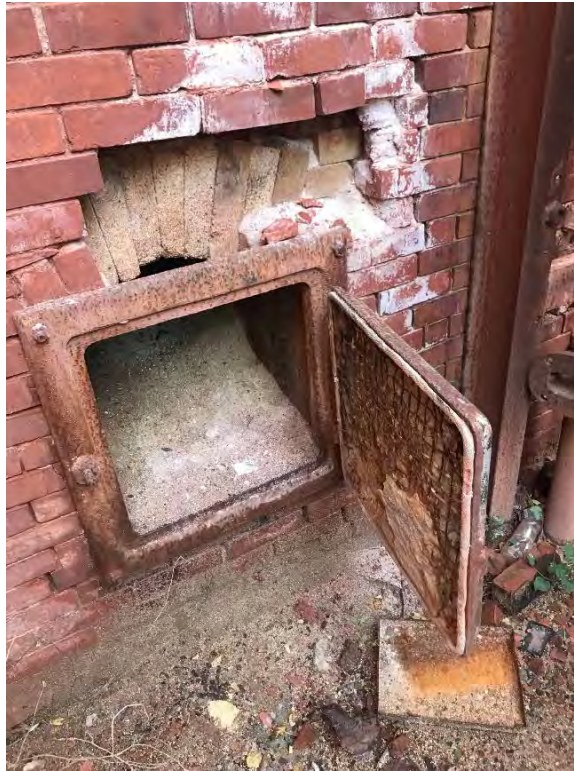
Boiler access doors showing asbestos containing rope gasket and cement on inside of door
