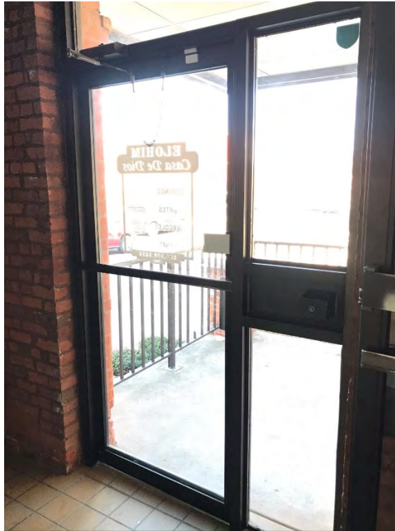
Type 3 Door: Dark gray caulking: Non asbestos, Presumed PCBs >50 PPM (same caulking on Type 5 Door); No glazing observed
