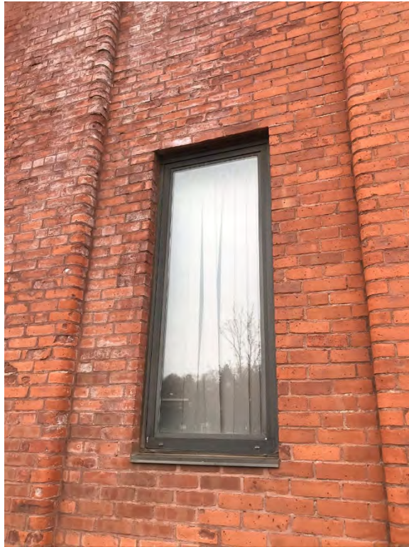
Type 1 Window: Gray caulking: Non asbestos, Presumed PCBs >50 PPM; No glazing observed
