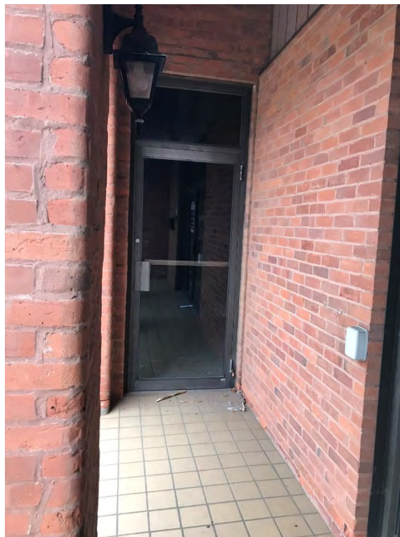
Type 2 Door: Brown caulking: Non asbestos, Presumed PCBs >50 PPM; No glazing observed
