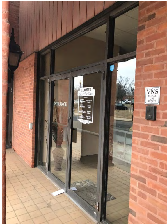
Type 1 Doors: No caulking or glazing observed
