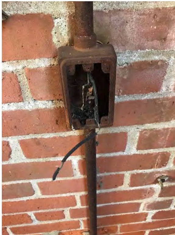
Example of asbestos containing electrical wire wrap
