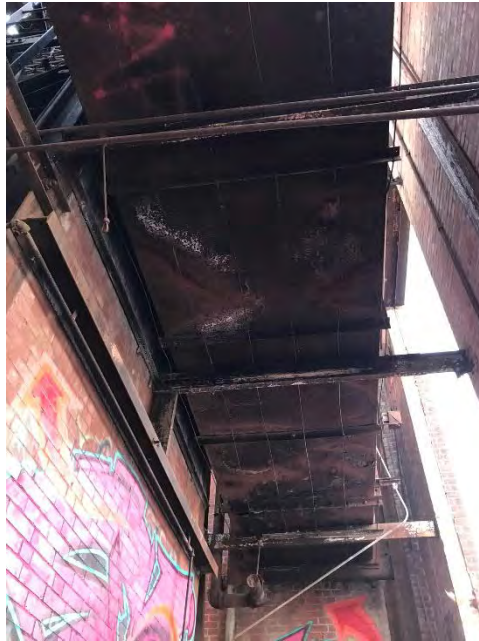
Duct attached to boilers. Seam sealant assumed present and if located should be presumed to contain asbestos.
