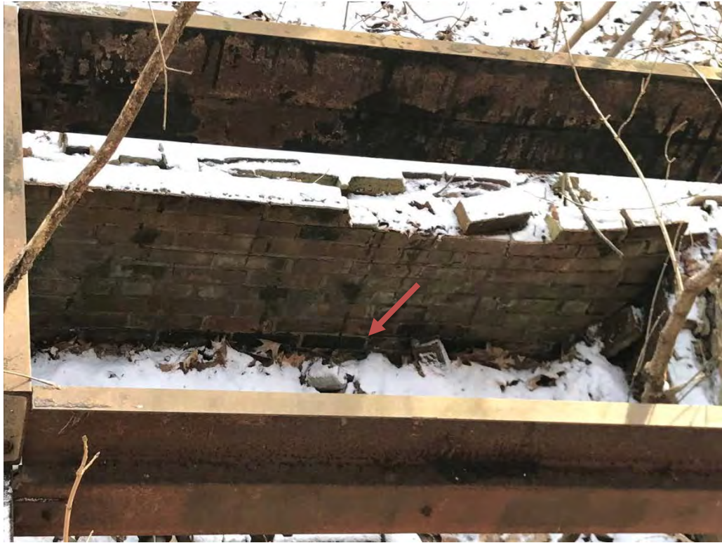
Black material observed on brick wall of vault. Material could not be inspected closely. May be waterproofing. Assumed asbestos containing.
