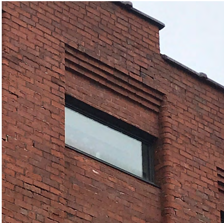
Type 4 Windows: Gray caulking: Non asbestos, Presumed PCBs >50 PPM; No glazing observed
