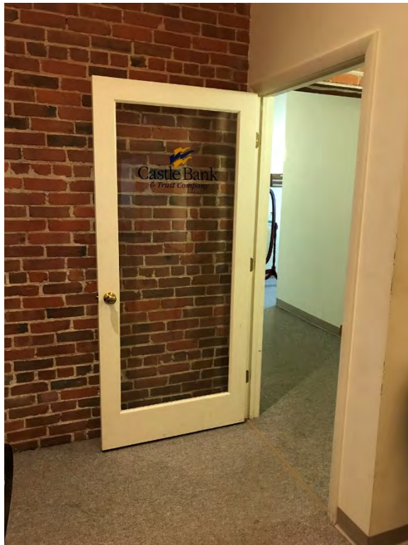
Type 10 Door: No caulking or glazing observed
