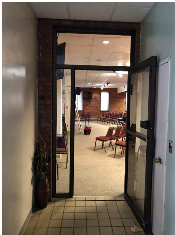
Type 6 Door: Dark brown caulking; 3% Asbestos, Presumed PCBs >50 PPM; No glazing observed
