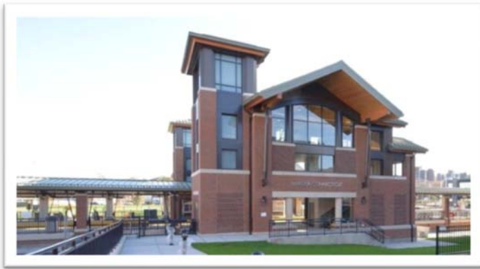
1 Meriden Transit Center
